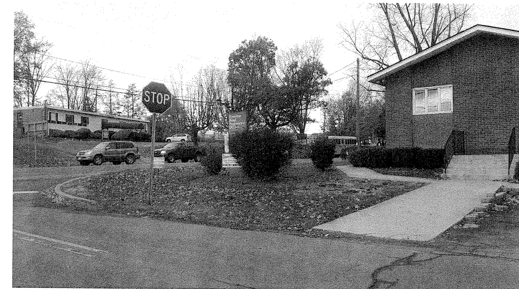
8 SITE PHOTO - CORNER EX-2
