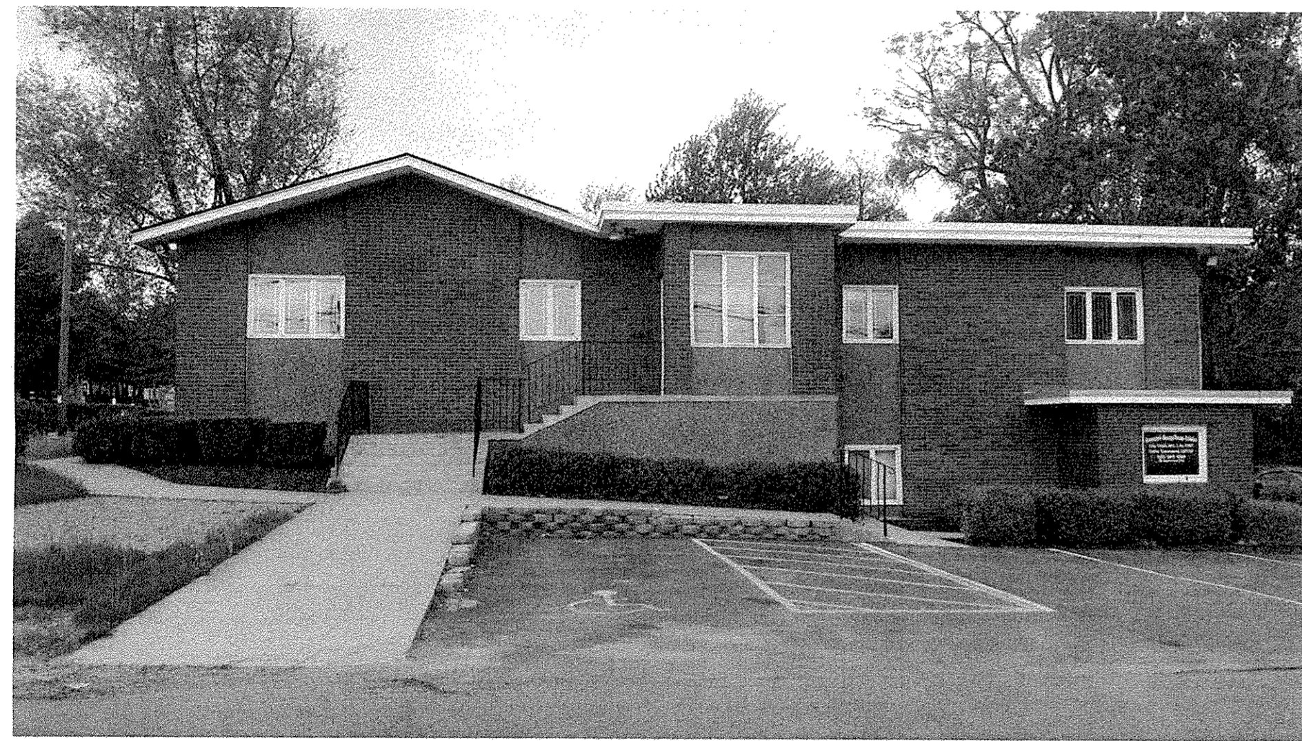
4 SITE PHOTO - EAST SIDE EX-2
