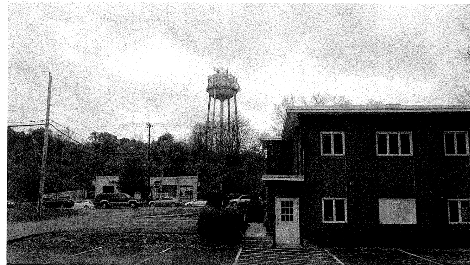
7 SITE PHOTO - SOUTH VIEW EX-2
