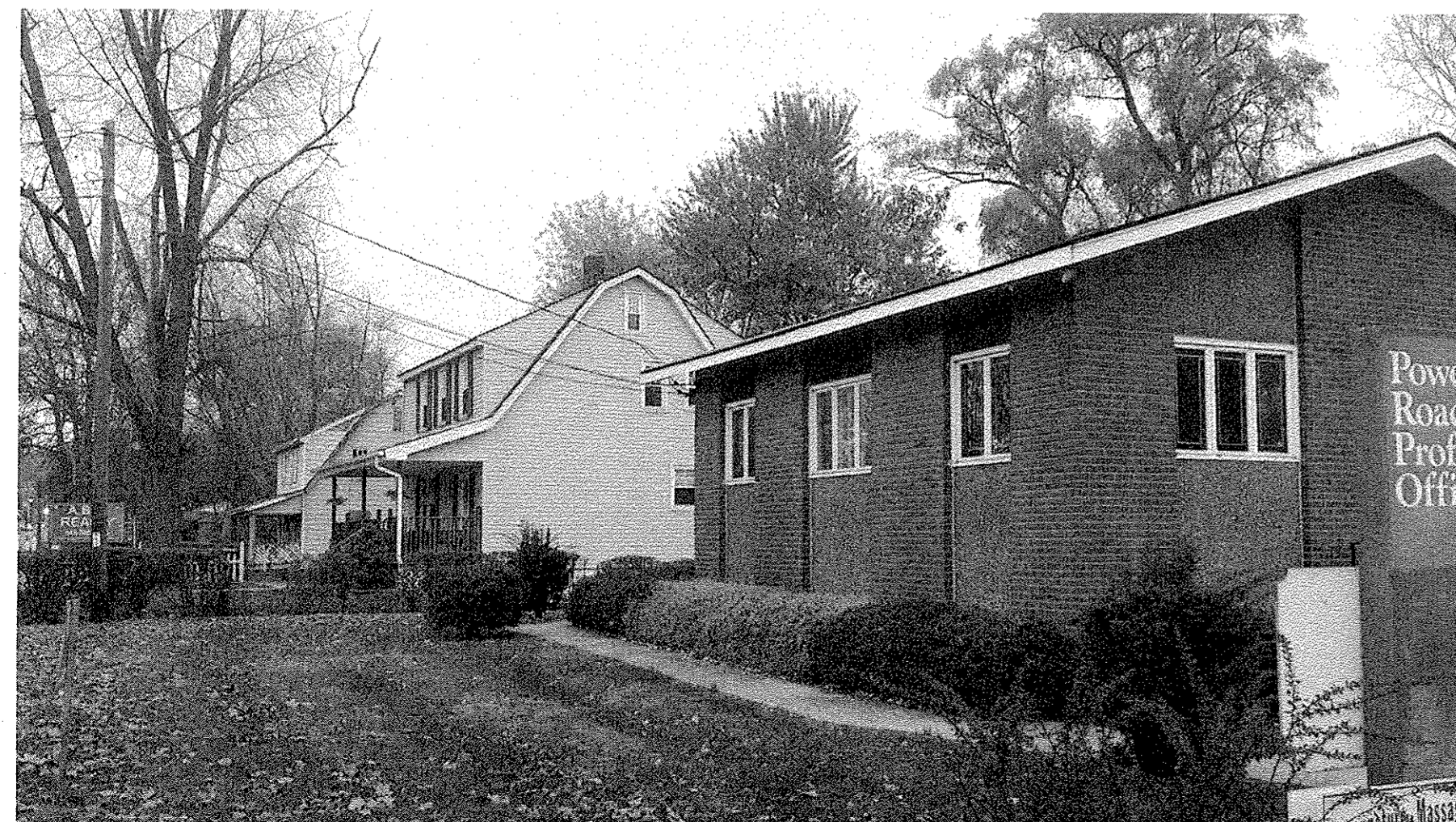
6 SITE PHOTO - NORTH PLANK ROAD EX-2
