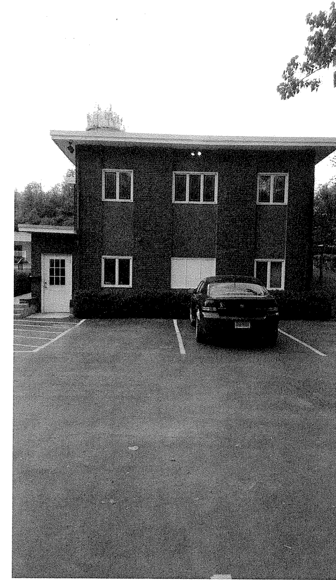
3 SITE PHOTO - NORTH SIDE EX-2
