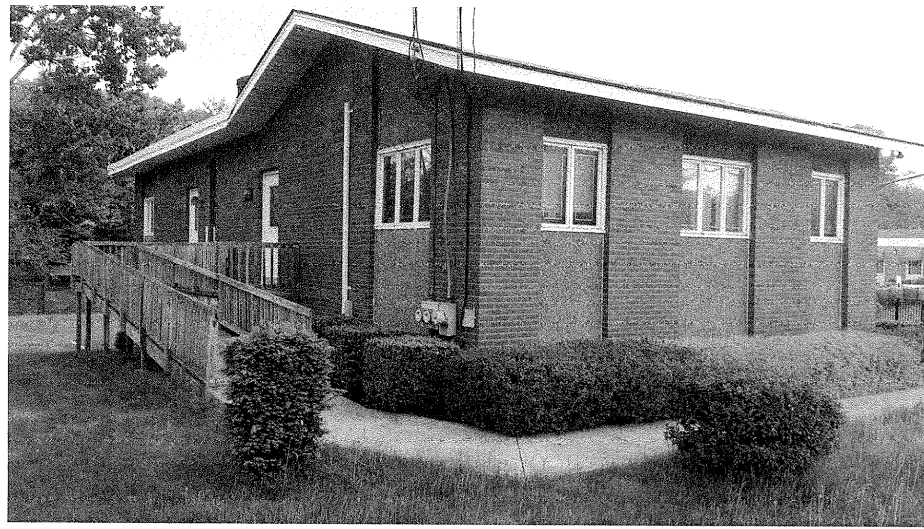
1 SITE PHOTO - SOUTH WEST SIDE EX-2
