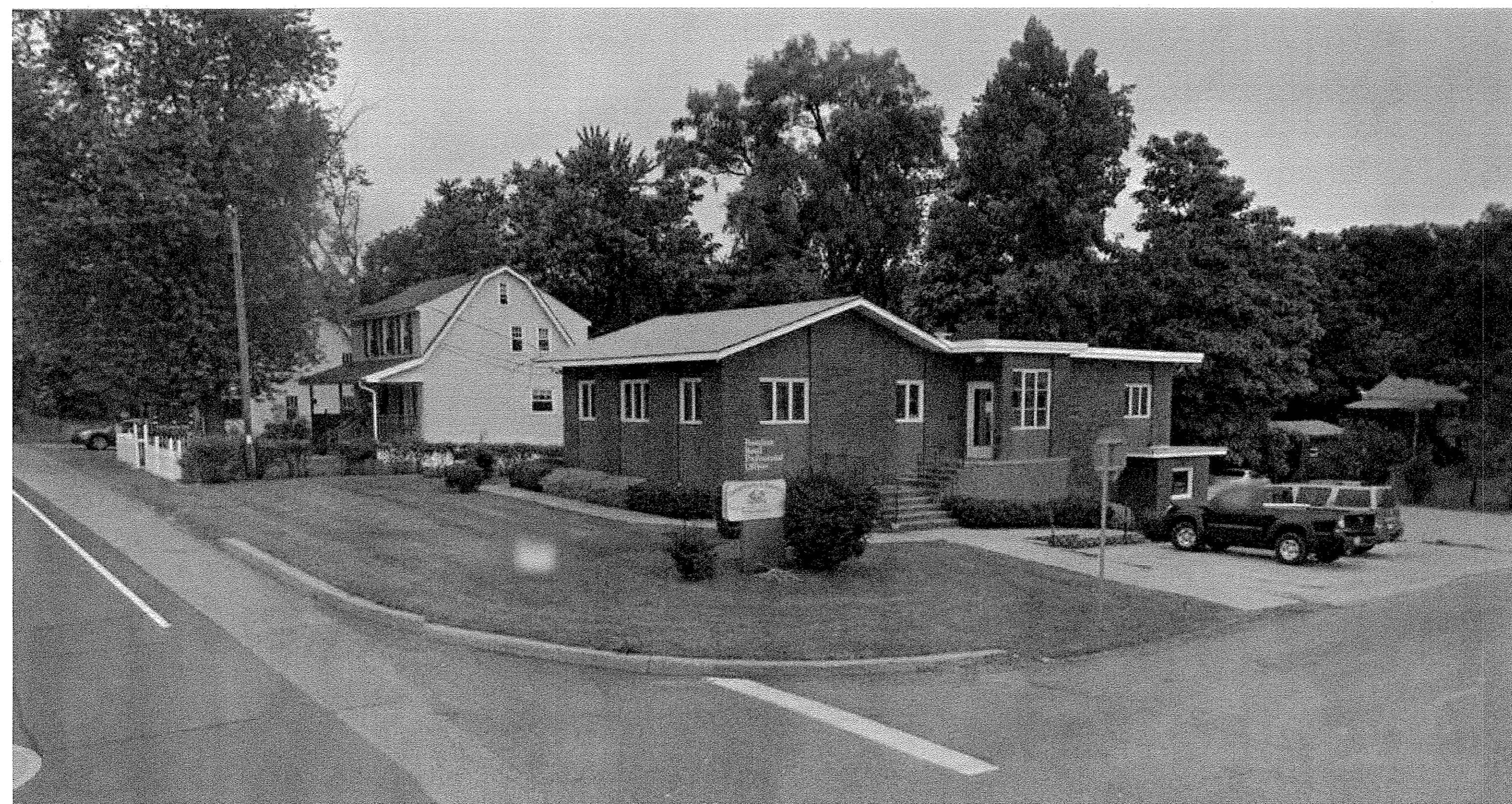
1 EXISTING NW VIEW EX-3
