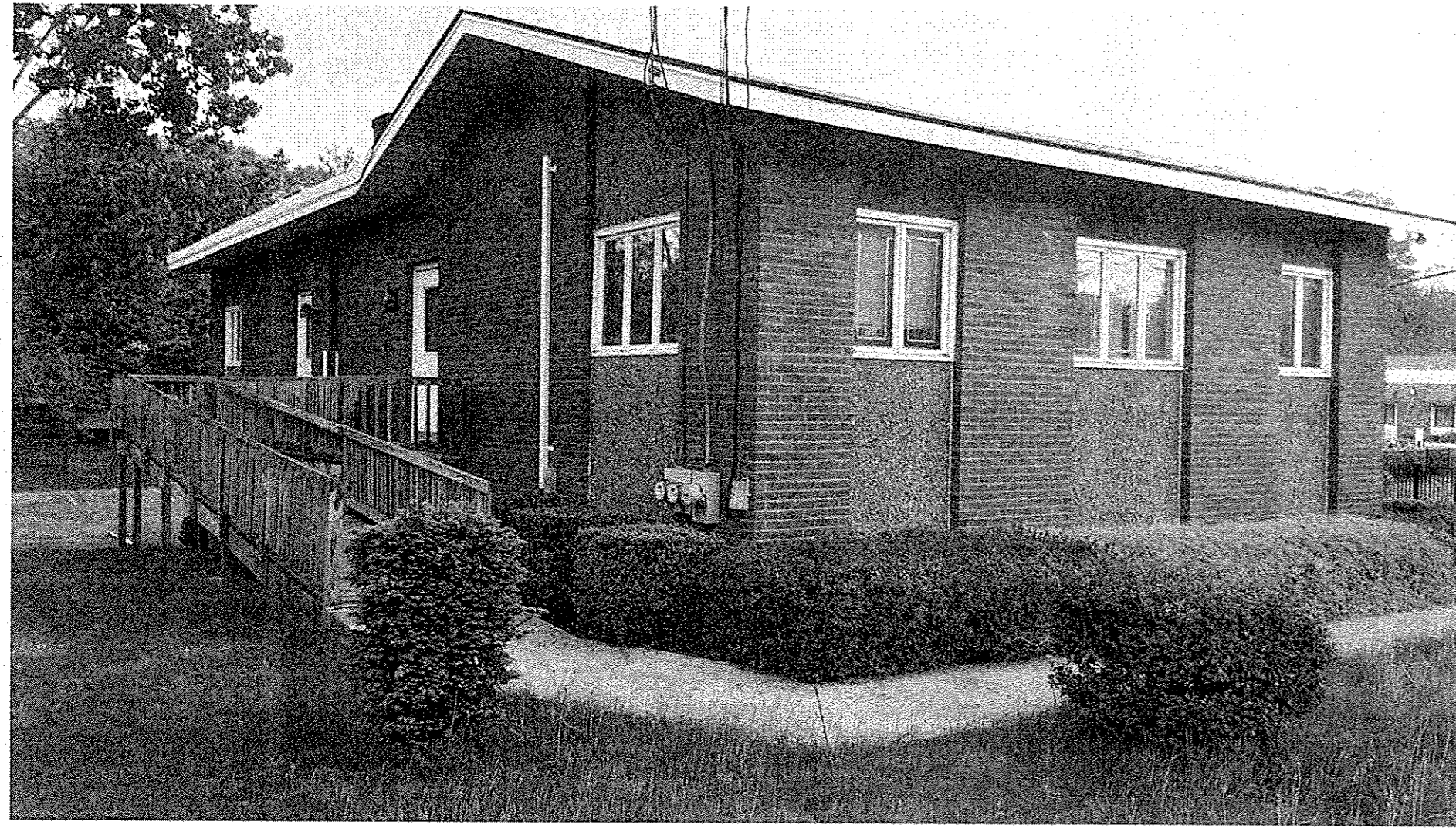
1 SITE PHOTO - SOUTH WEST SIDE EX-2
