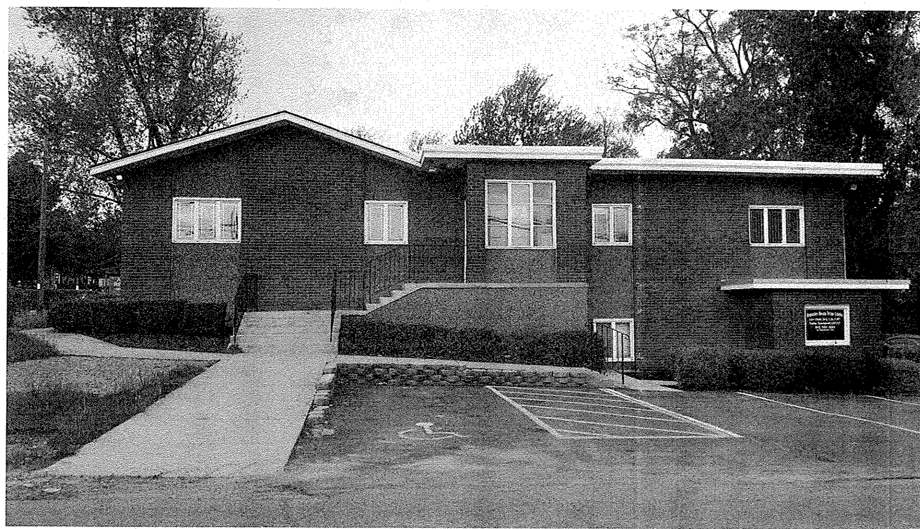
4 SITE PHOTO - EAST SIDE EX-2
