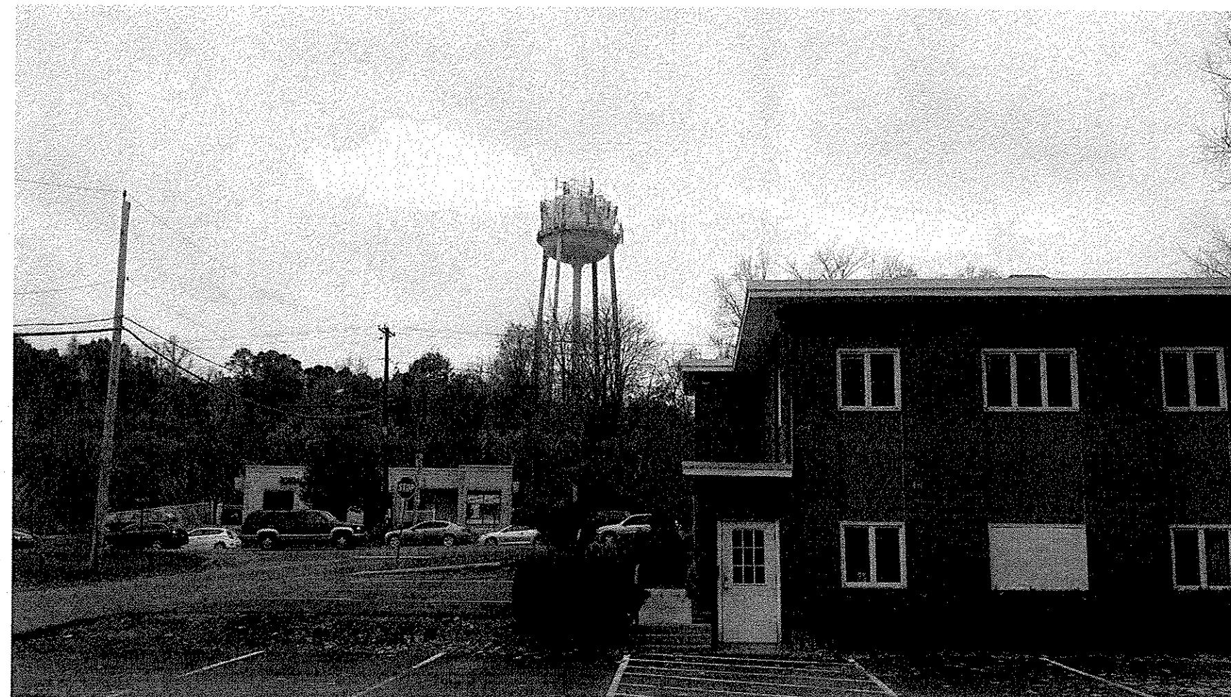
7 SITE PHOTO - SOUTH VIEW EX-2
