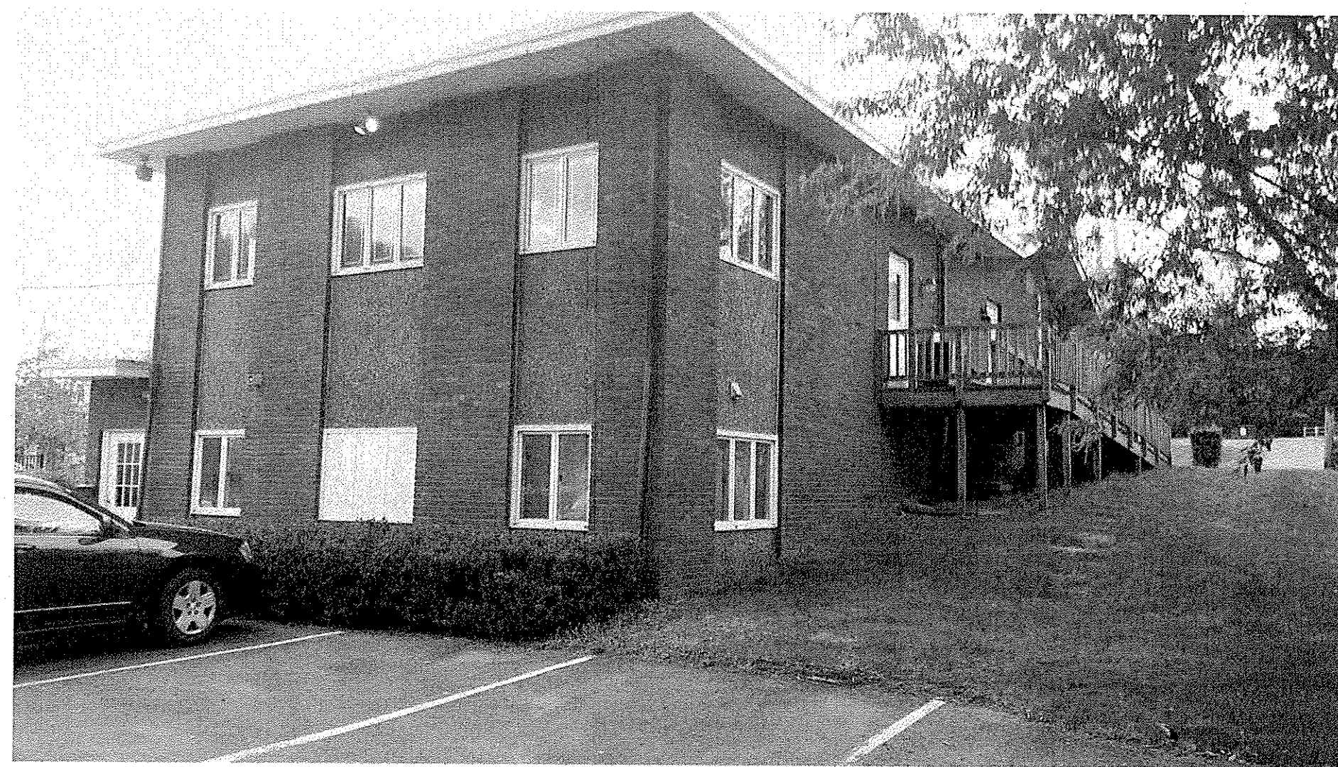
2 SITE PHOTO - NORTH WEST SIDE EX-2
