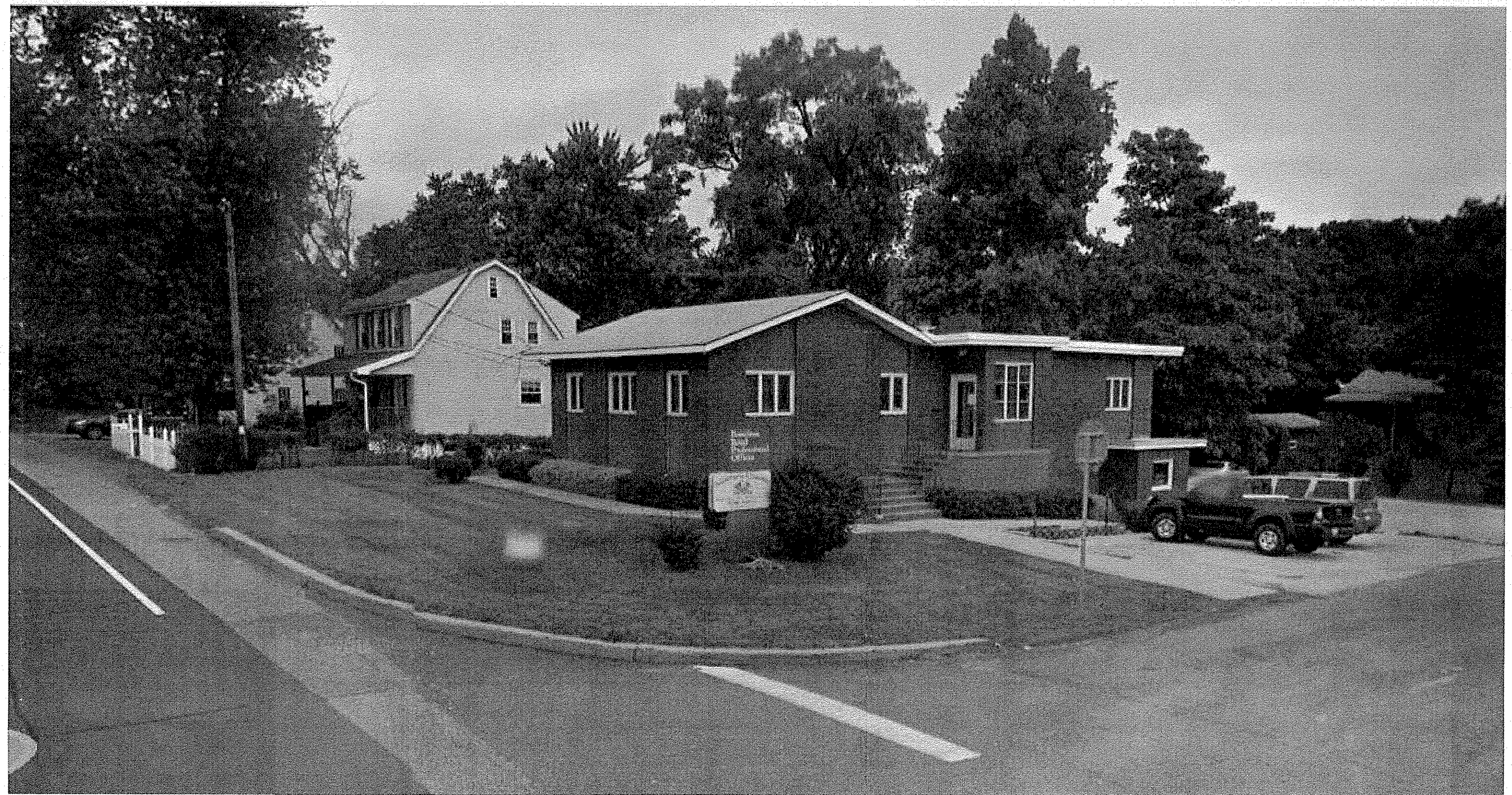
1 EXISTING NW VIEW EX-3
