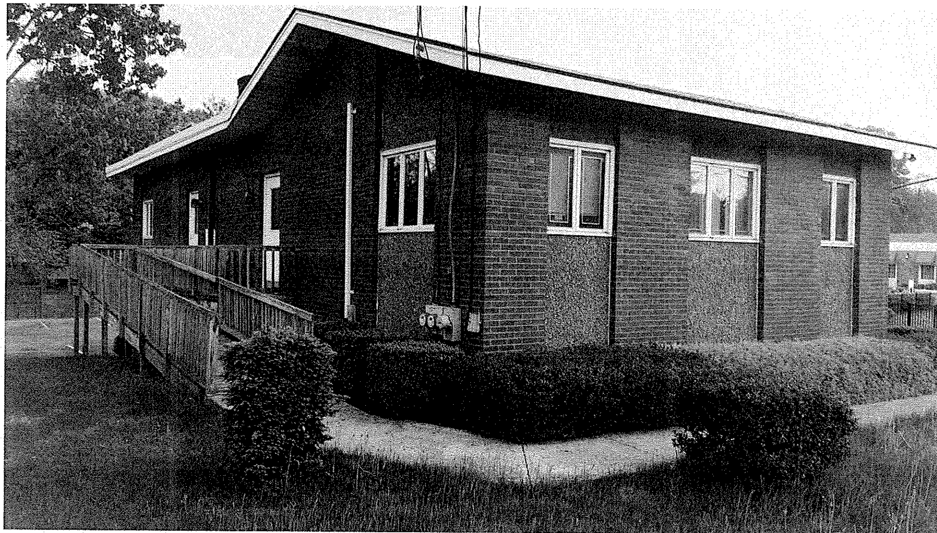
1 SITE PHOTO - SOUTH WEST SIDE EX-2
