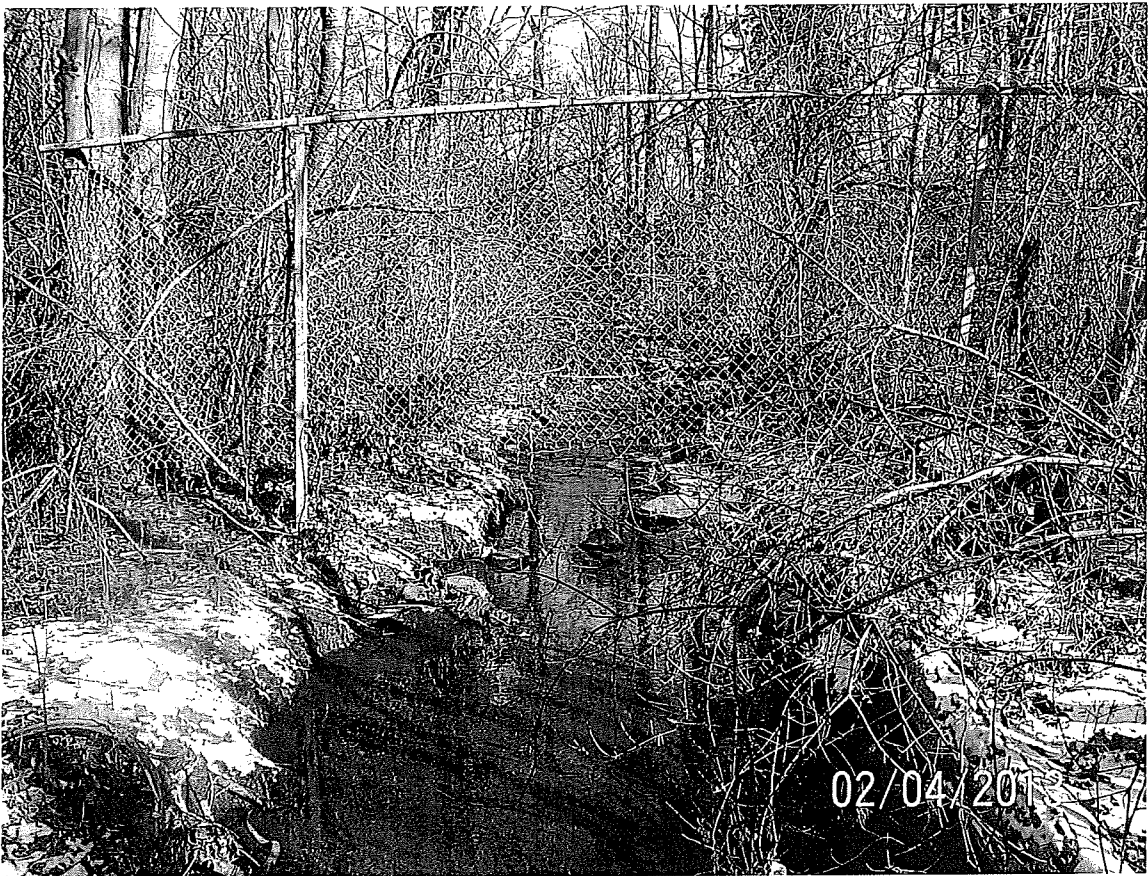
Photo 7 –View north of Route I-84 Culvert
