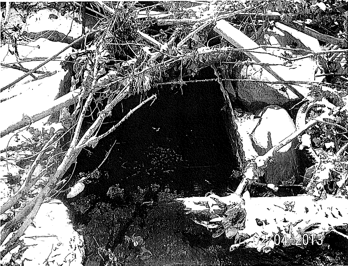
Photo 6 -Route I-84 Culvert
