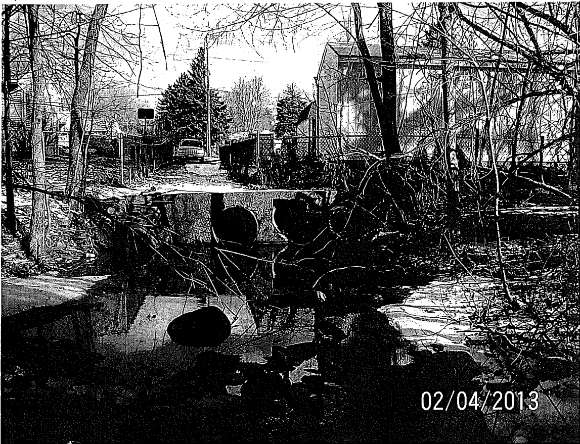
Photo 8 –Meadow Hill Drainage Discharge
