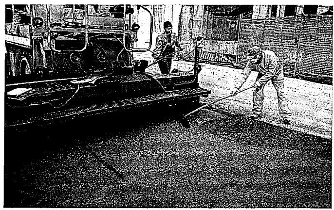
Paving operations should be conducted in dry weather.
