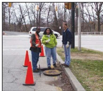
Figure 54: Traffic cones divert traffic from manhole inspection area
