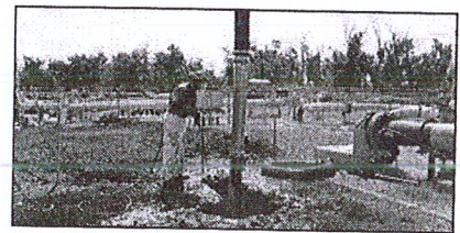
Hydro Excavation in the Oil Industry
